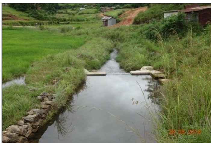
Figure-72: Field Photograph of Water Harvesting Structures
